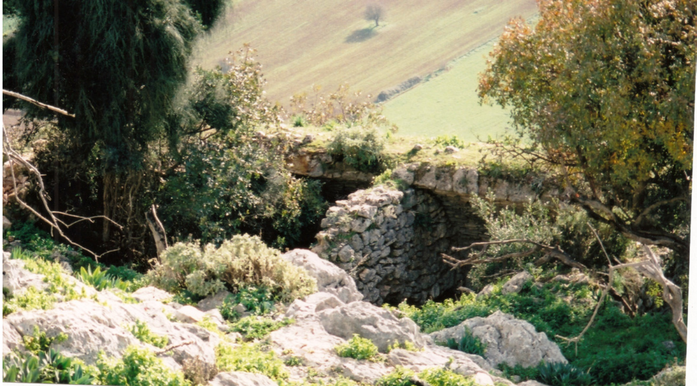
Fig. 29. Castle of Aetos. Cistern.
